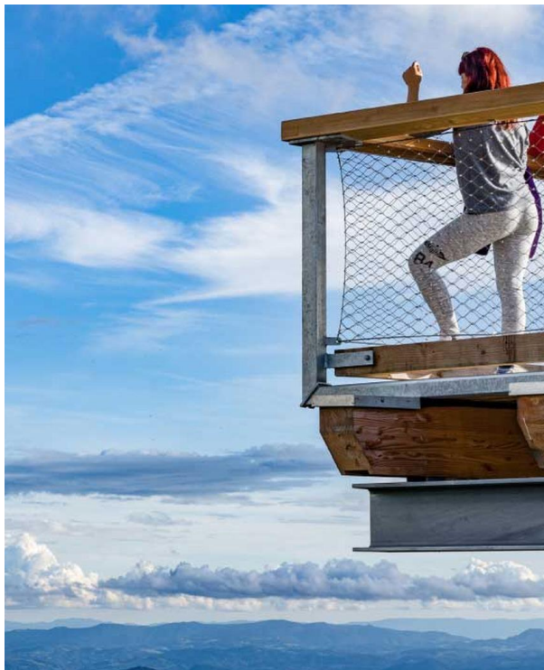
The 37-metre lookout tower
