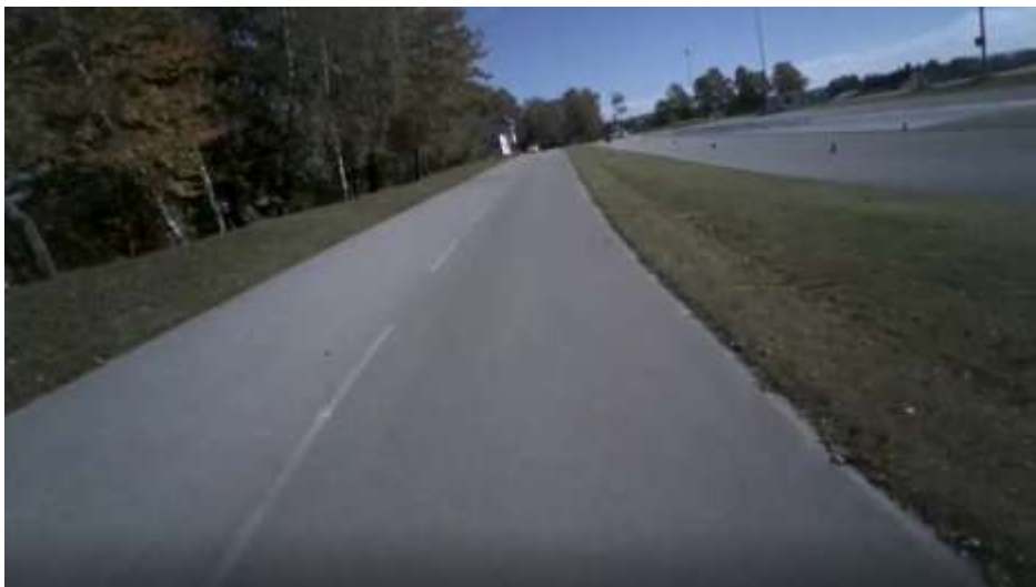
Figure 9: Straight stretch of road – second part
