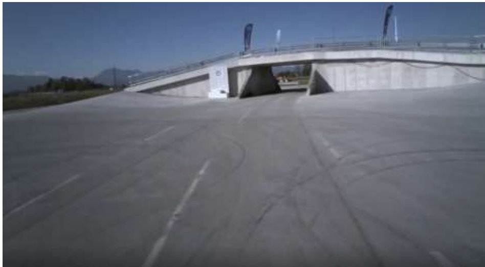
Figure 5: Through an underpass
