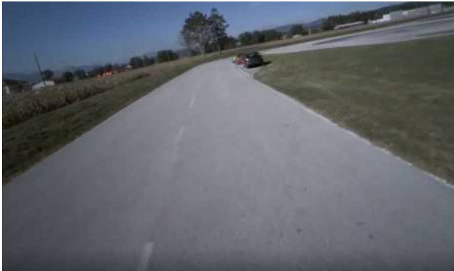
Figure 8: Straight stretch of road – first part
